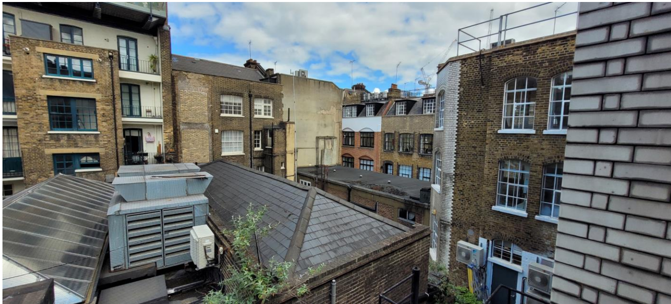
View towards rear/ flat roof of 9 -11 Langley Court
